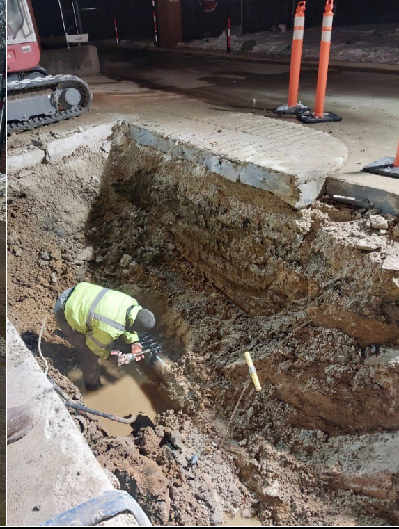
Repair Clamp Being Installed
