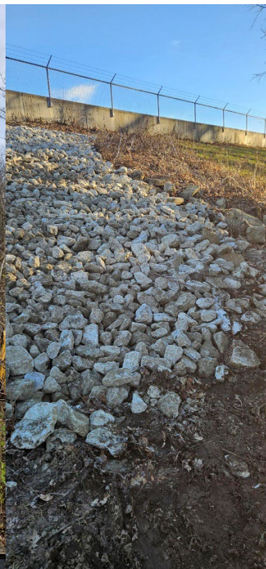
South Levee Wall – After Clearing and Rip Rap Installation
