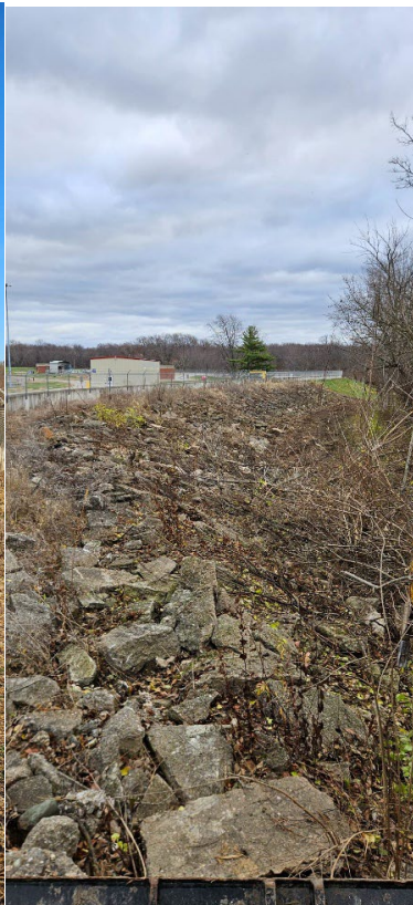
South Levee Wall – After Clearing and Rip Rap Installation
