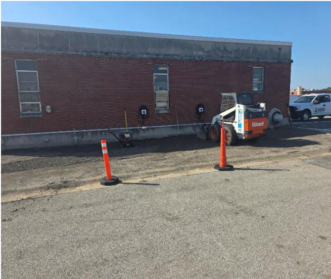
EV Parking Area
