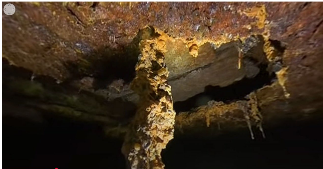
Image of hole in Secondary Digester #2 lid
