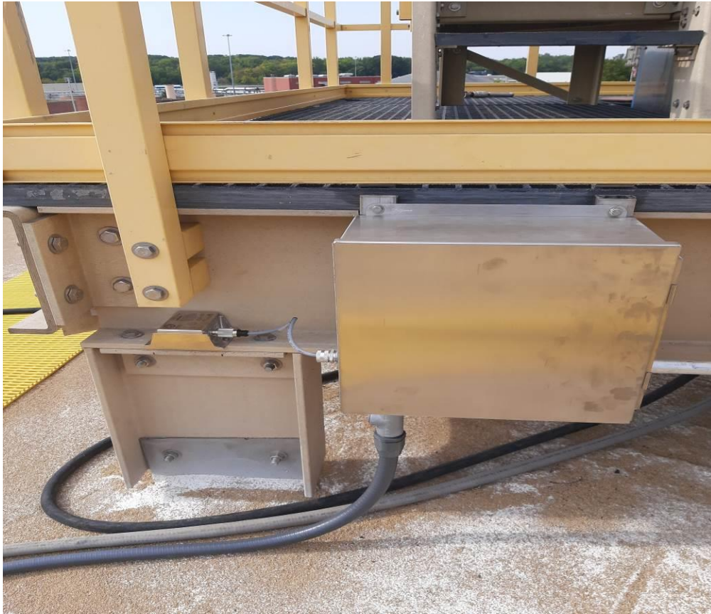
Digester #3 Lid Level Inclinometer Installation
