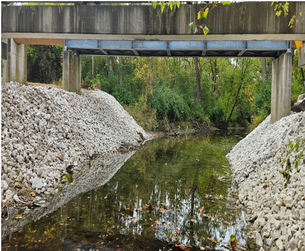
Stevens Creek Trestle – Looking South – After –
