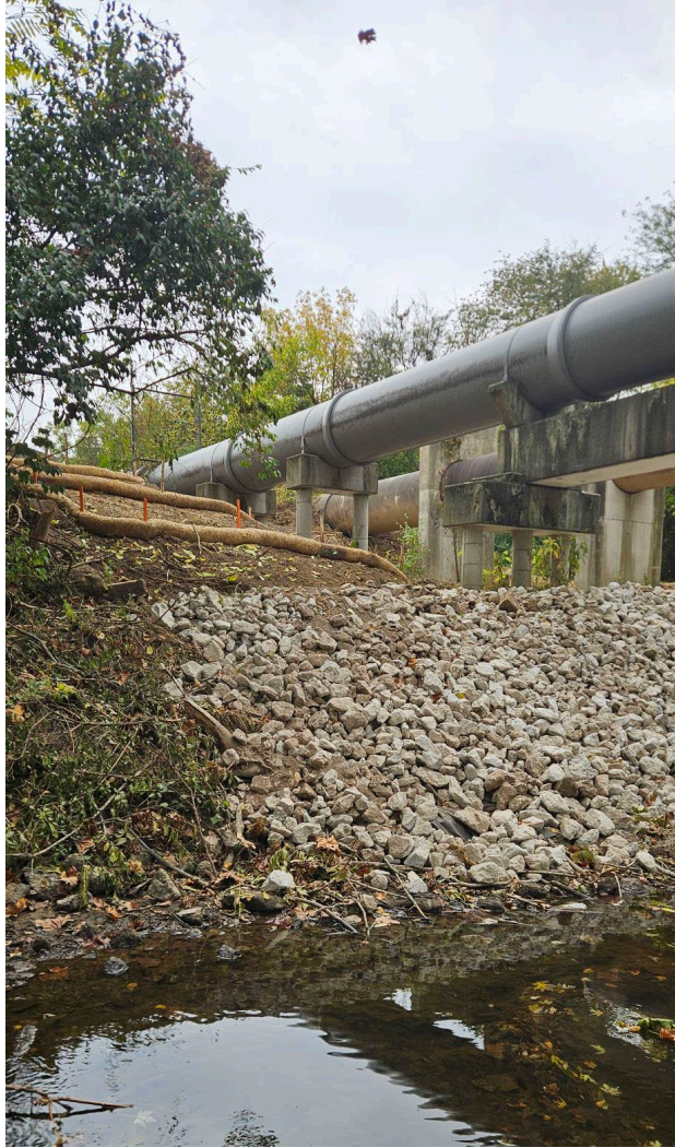
Stevens Creek Trestle – Looking East – After
