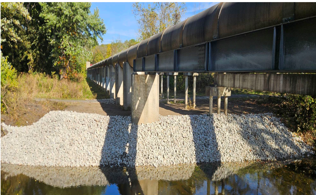
Stevens Creek Trestle – Looking West - After
